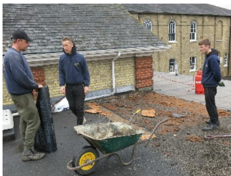
Flat roof repairs
