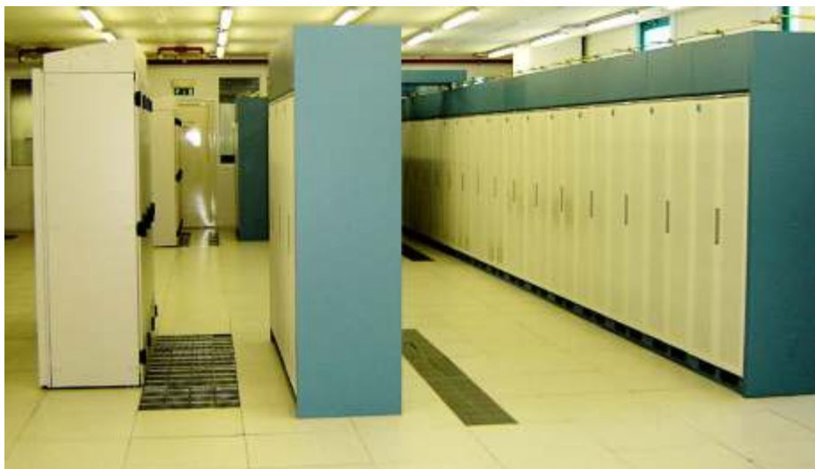
Lucent 5ESS used in a mobile network [PD]
