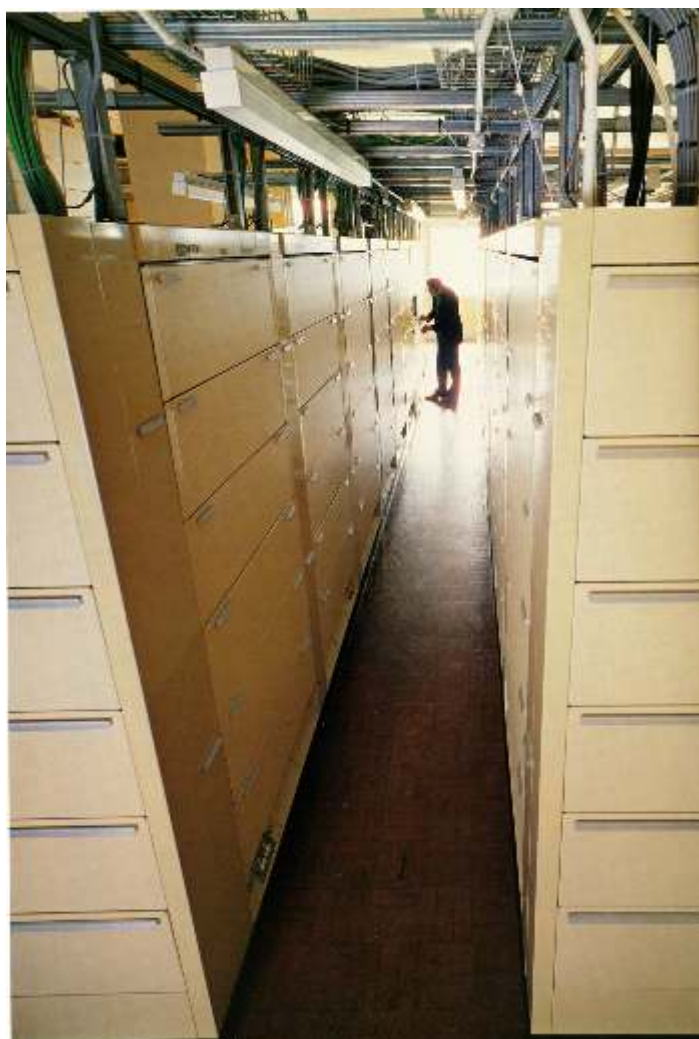
Typical System X exchange [BT]
