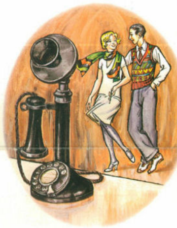
Called 'candlestick' telephones because of their shape, these were used from the 1880's for over half a century. Later models had dials. 1905
