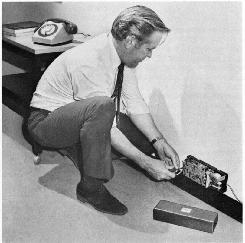
Installing a subscriber terminal unit
