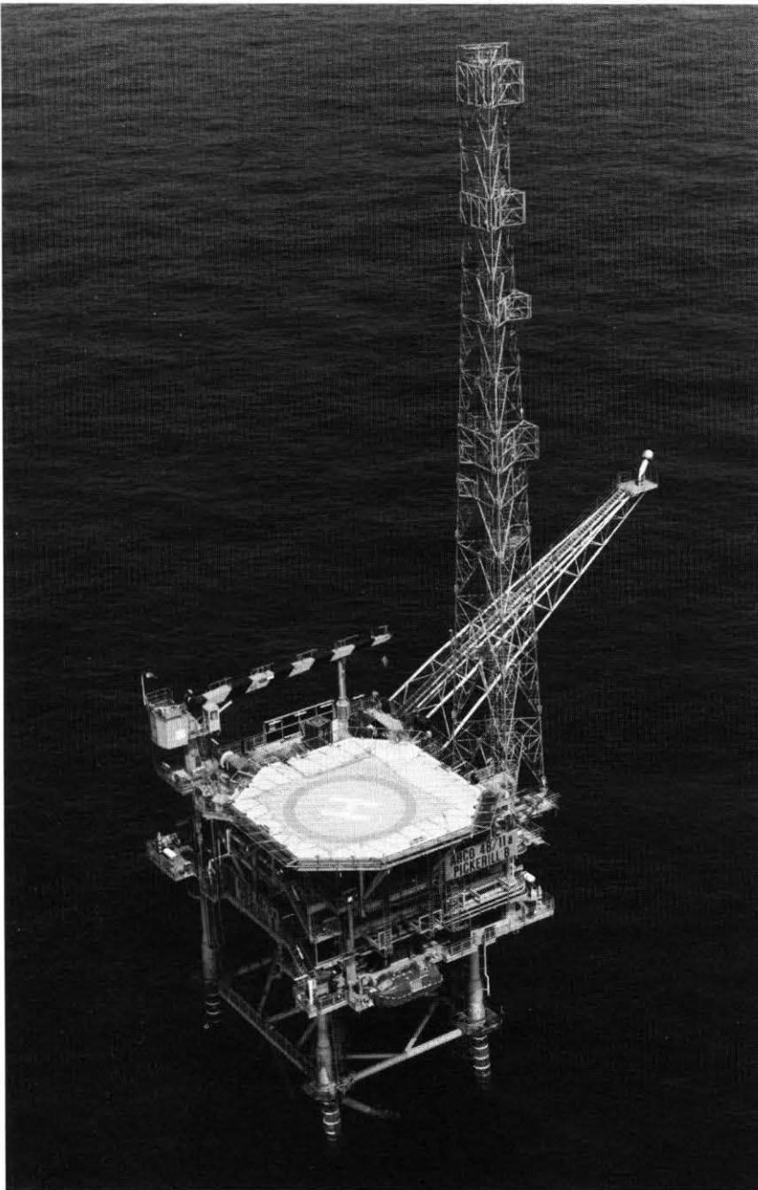
Figure 6—Pickerill B platform
