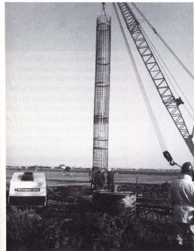
Figure 3—Onshore mast foundations under construction
