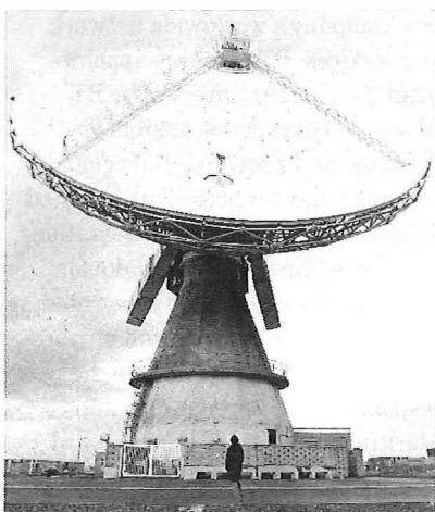
Goonhilly satellite earth station
