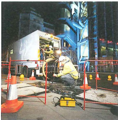
BT cable laying in the City of London
