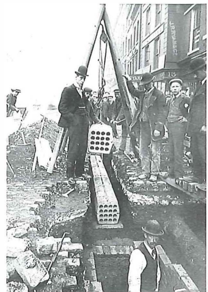
Laying ducts in the early years of telecommunications
