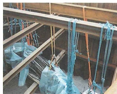
Figure 2—Temporary support of existing BT cables
