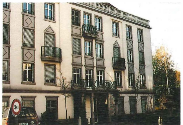
Figure 10—Old building in Dubendorf
