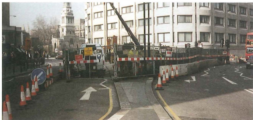
Figure 1—Typical city centre site showing traffic diversions, protection and fencing off
