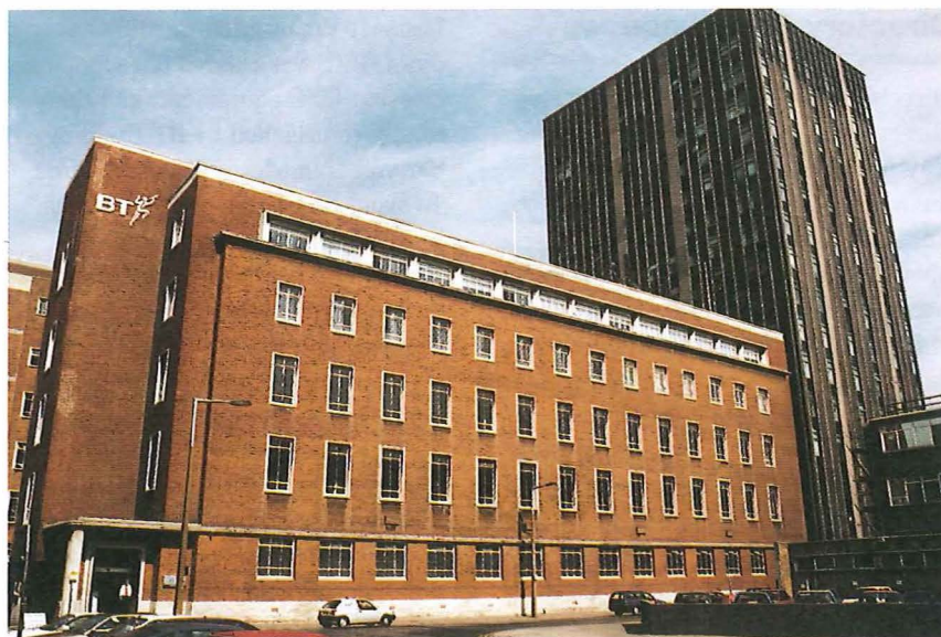
Figure 1 – Cardiff Empire exchange (Stadium House is on the right)
