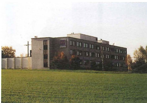
Figure 9—New building in Rumlang
