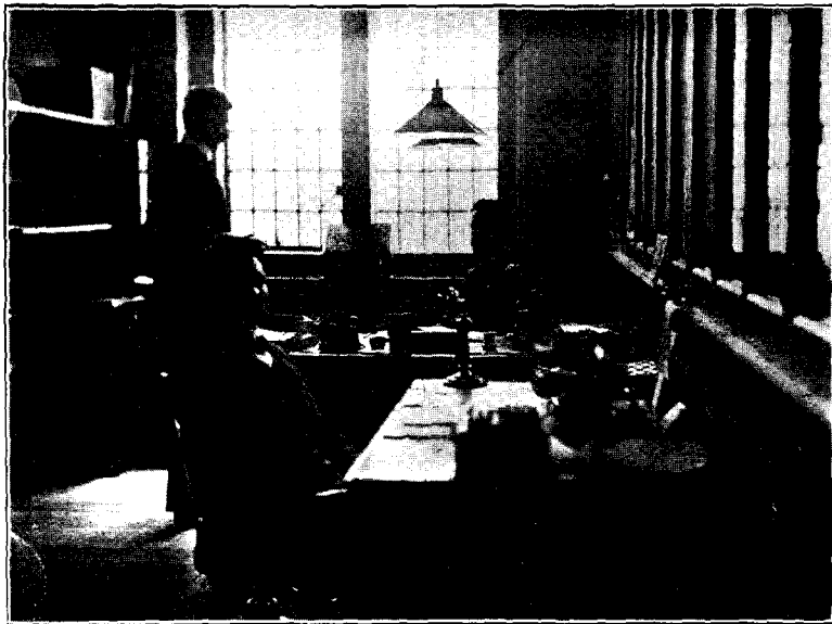
FIG. 2. - EXCHANGE ELECTRICIAN'S OFFICE, GERRARD.
