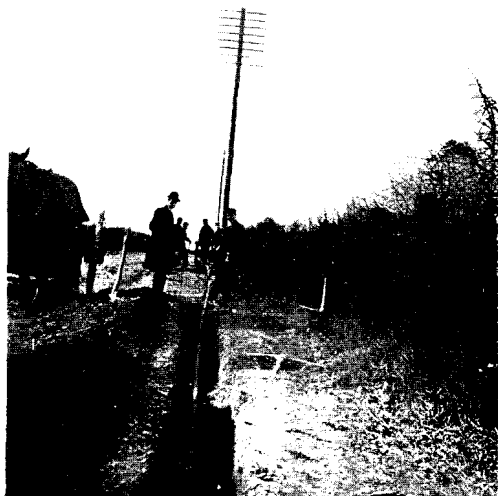
USING THE SPRING BALANCE IN SERIES WITH THE HAULING ROPE.
