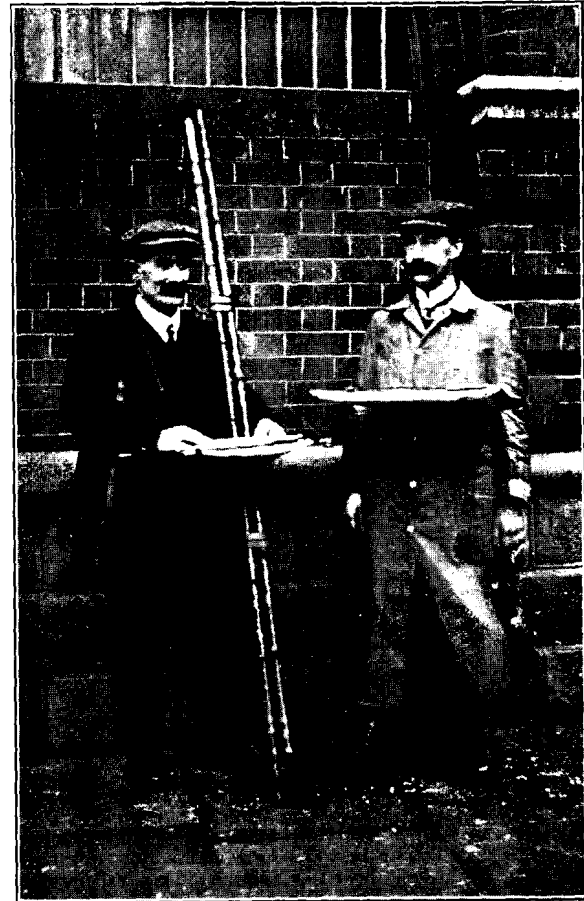
OVERHEAD AND UNDERGROUND ENUMERATORS, A AND C DIVISIONS.
