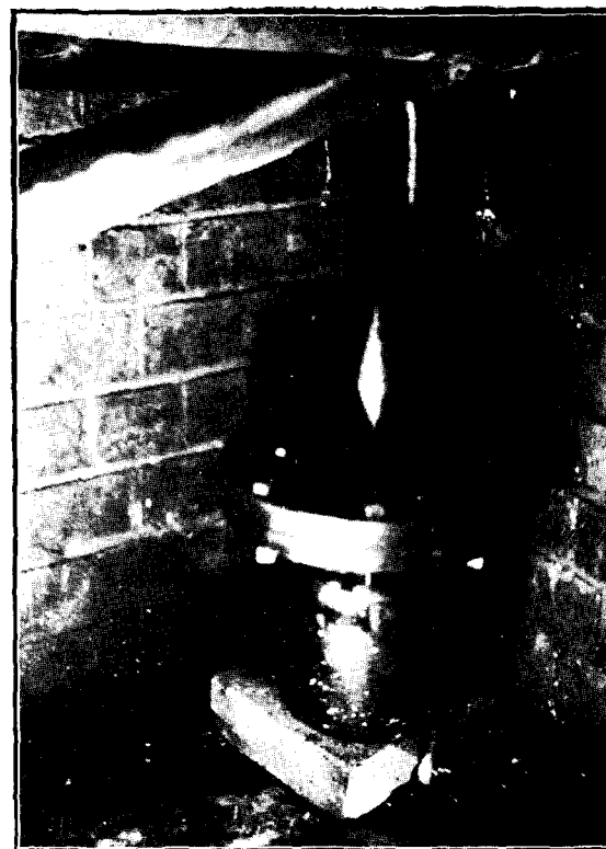
FIG. 5.—View of Coil Pot on Floor of Manhole before Iron Band was Fitted.
