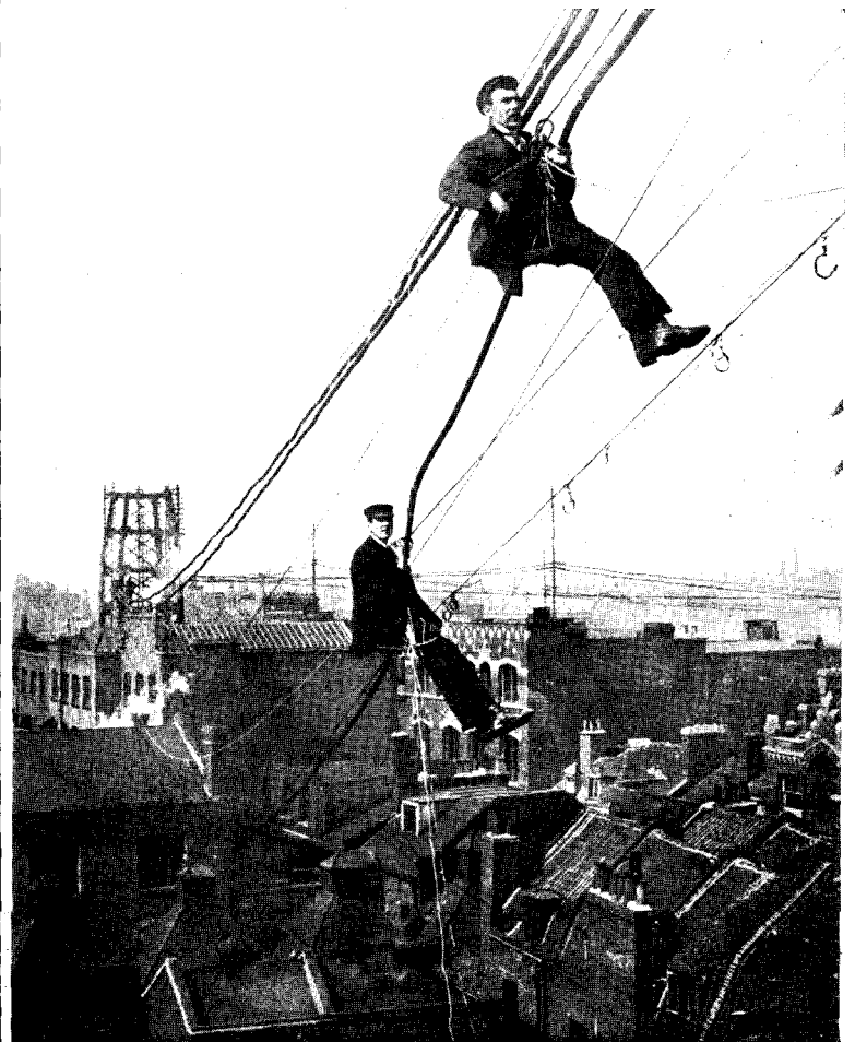
OVERHOUSE TELEPHONE CONSTRUCTION.
