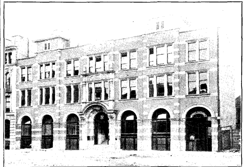
BRISTOL EXCHANGE - BALDWIN STREET. (Faced with red bricks and dressings of Bath Stone.)
