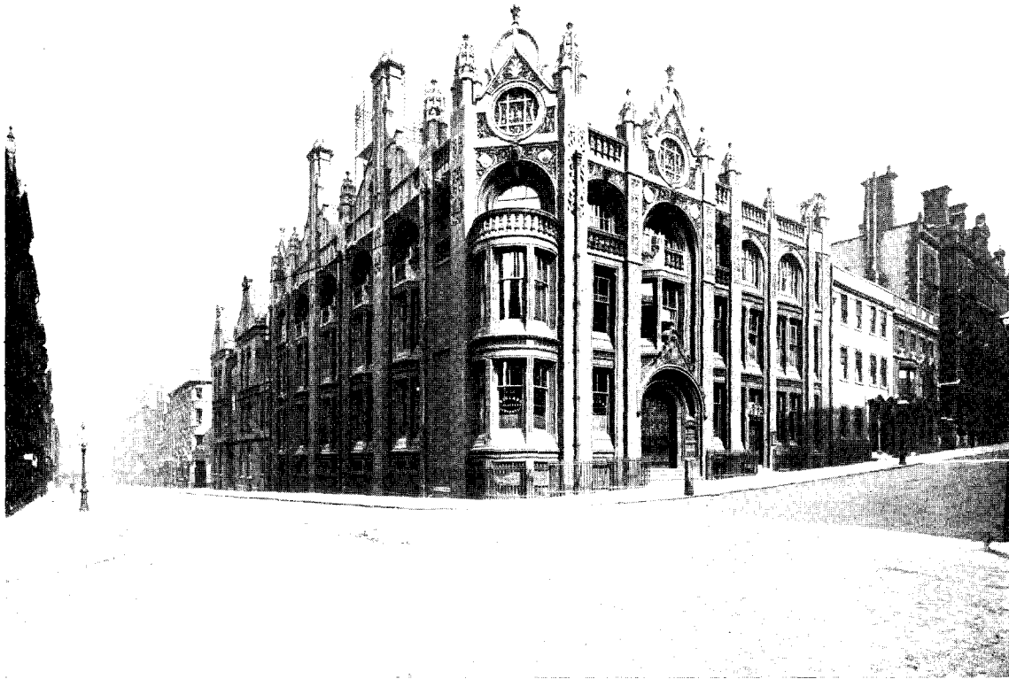
BIRMINGHAM CENTRAL EXCHANGE—NEWHALL STREET. (Faced with Ruabon red bricks and terra-cotta dressings.)
