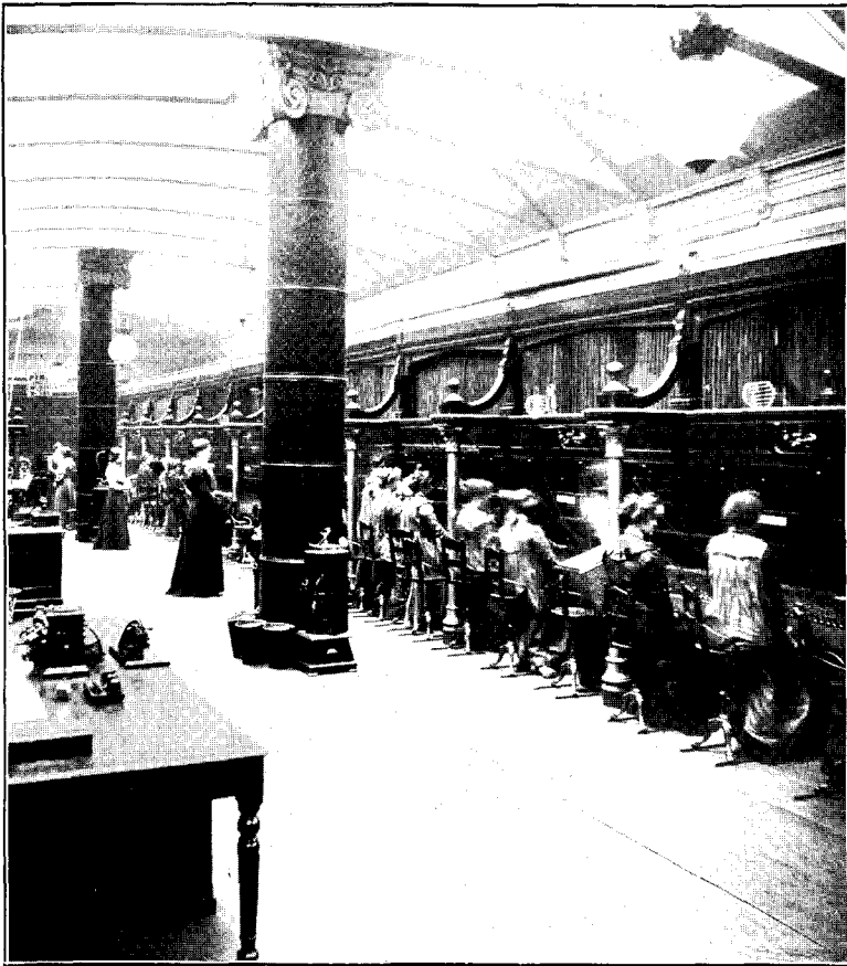
FLAT MULTIPLE SWITCHBOARD—GLASGOW EXCHANGE, 1893.
