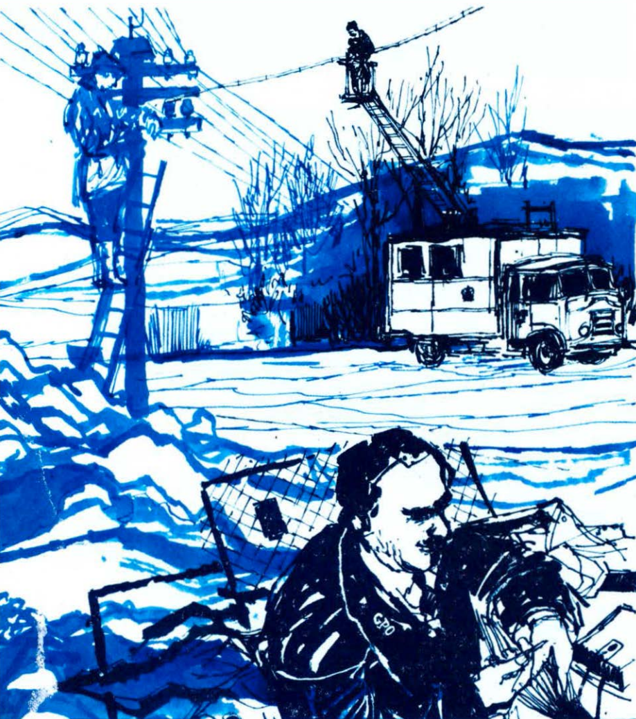
Left: The linesman's job is a tough one—above ground or below, in a howling gale or ten degrees of frost, the lines must be kept in good order.
