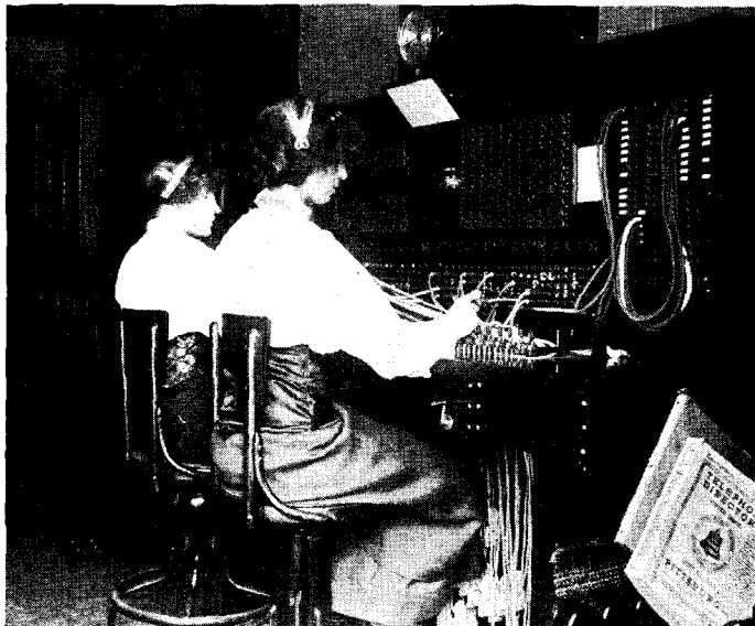
FIG. 4.—SWITCHBOARD PROVIDED WITH TEST PANEL.
