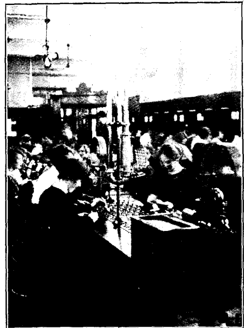
PNEUMATIC TICKET DISTRIBUTION.
