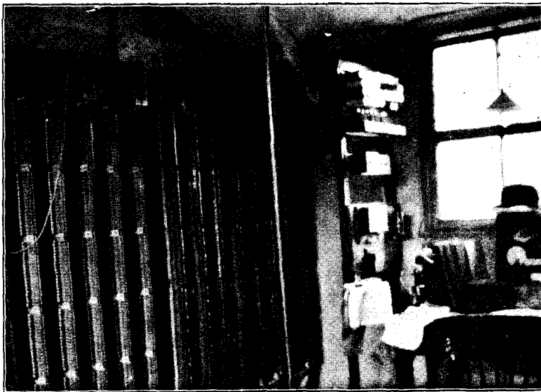
BROADWAY EXCHANGE—APPARATUS ROOM.
