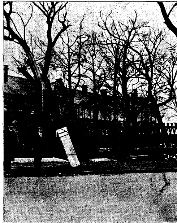
A LINE FAULT.
