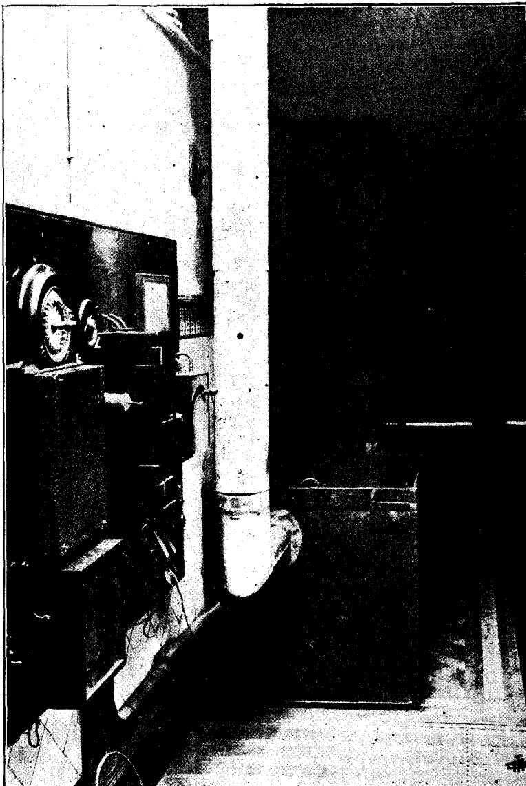
FIG. 8.—BANK EXCHANGE. THE POWER ROOM.
