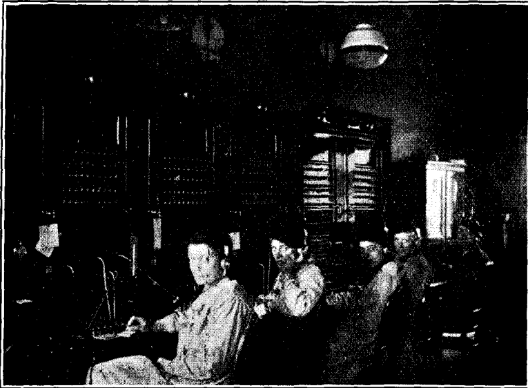
TRUNK EXCHANGE, S'HERTOGENBOSCH (MAGNETO MULTIPLE) 80 LINES 18 TELEPHONISTS IN BUSY HOURS (9—12).
