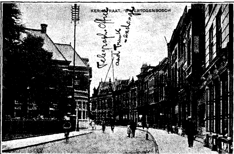
TELEPHONE OFFICE AND TRUNK EXCHANGE, S'HERTOGENBOSCH.
