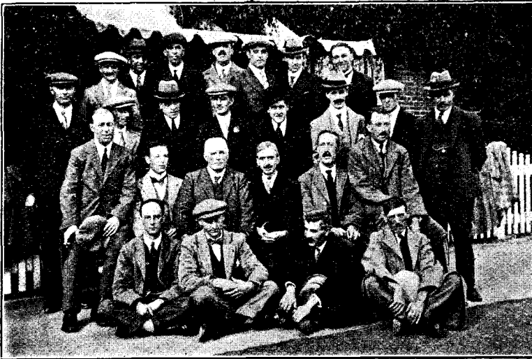
CABLE BALANCING STAFF OUTING.
