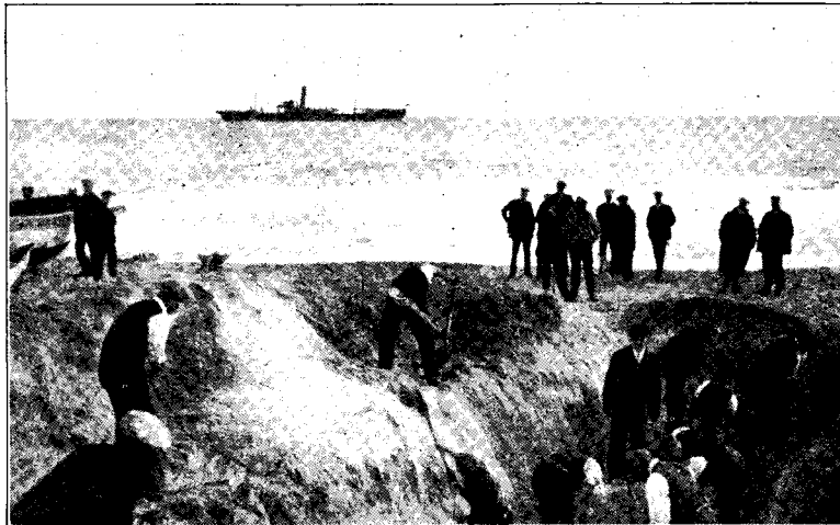
GERMAN CABLE STEAMER "STEPHAN" LAYING THE SHORE END OF THE MUNDSELEY-NORDENEY CABLE 1913.
