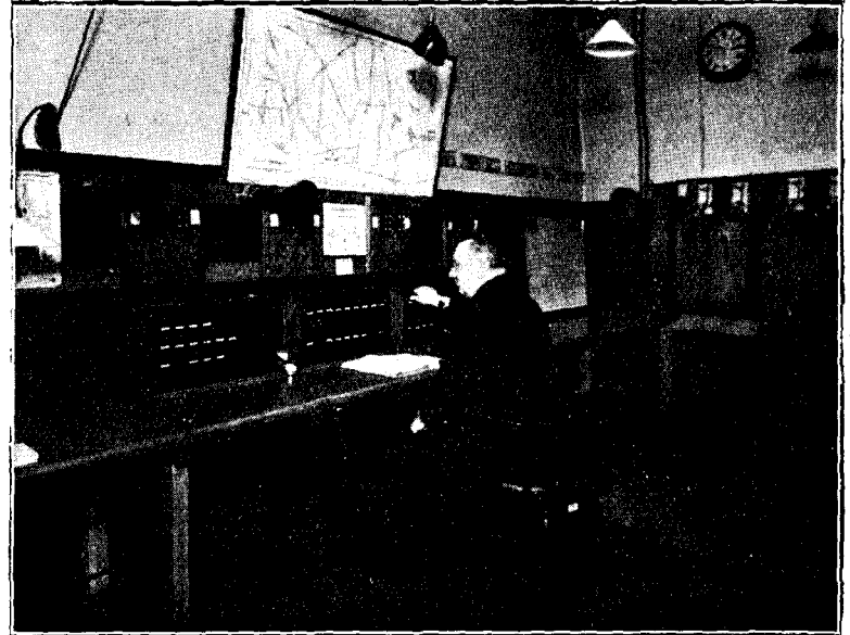
CONTROL ROOM, HACKNEY.
