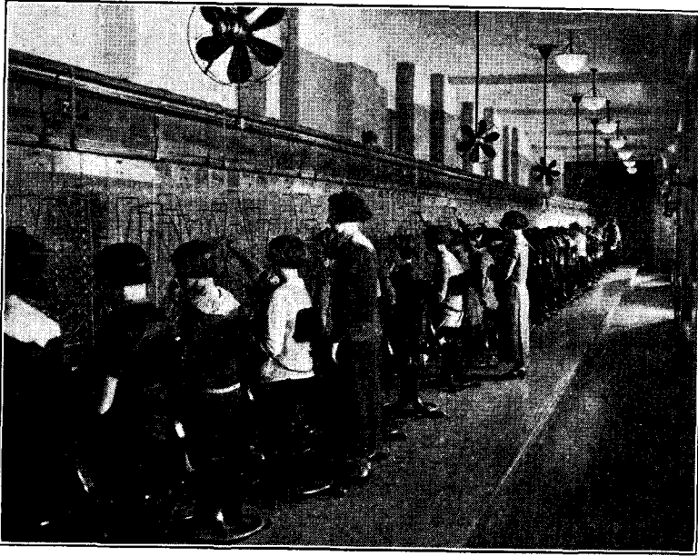
Interior of Los Angeles Telephone Exchange which figures in the film.
