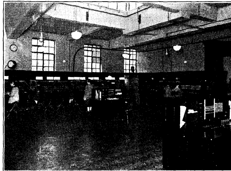
FIG. 1. GENERAL VIEW OF MANUAL SWITCHROOM.
