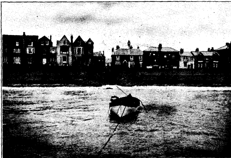
THE CABLE-END LANDED AT ALDEBURGH.
