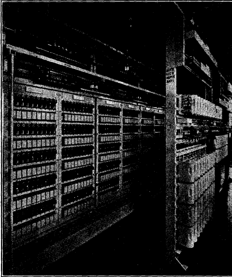
SHERWOOD EXCHANGE.—LINESWITCH UNITS AND REPEATER RACK.
