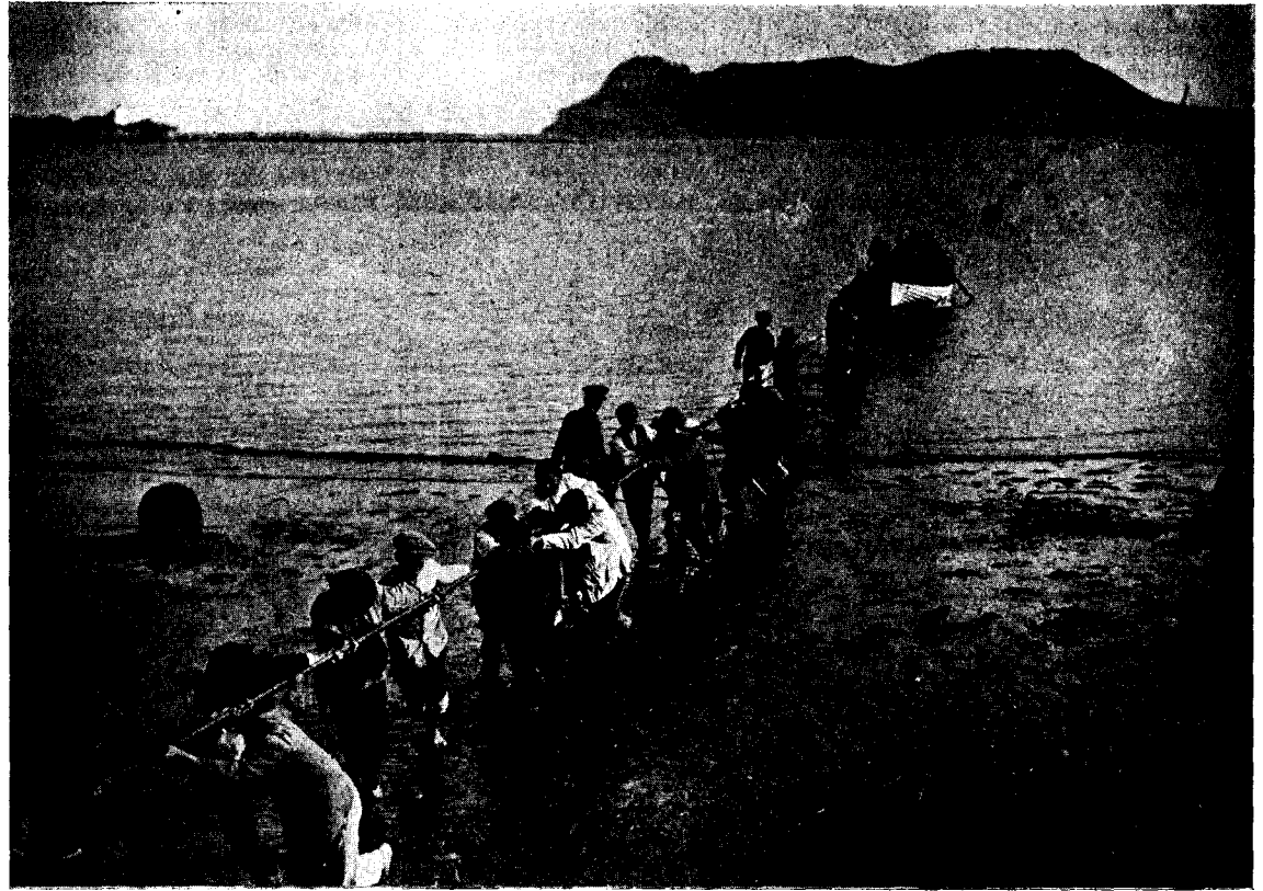
Landing the submarine telephone cable that unites Africa with Europe on the beach at Algeiras. The Rock of Gibraltar may be seen in the background.
