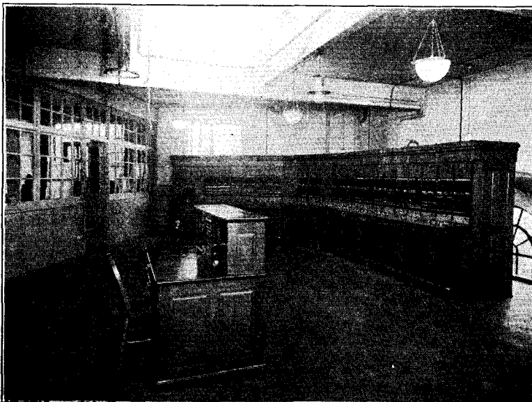
MANUAL BOARD WITH SUPERVISOR'S DESK.
