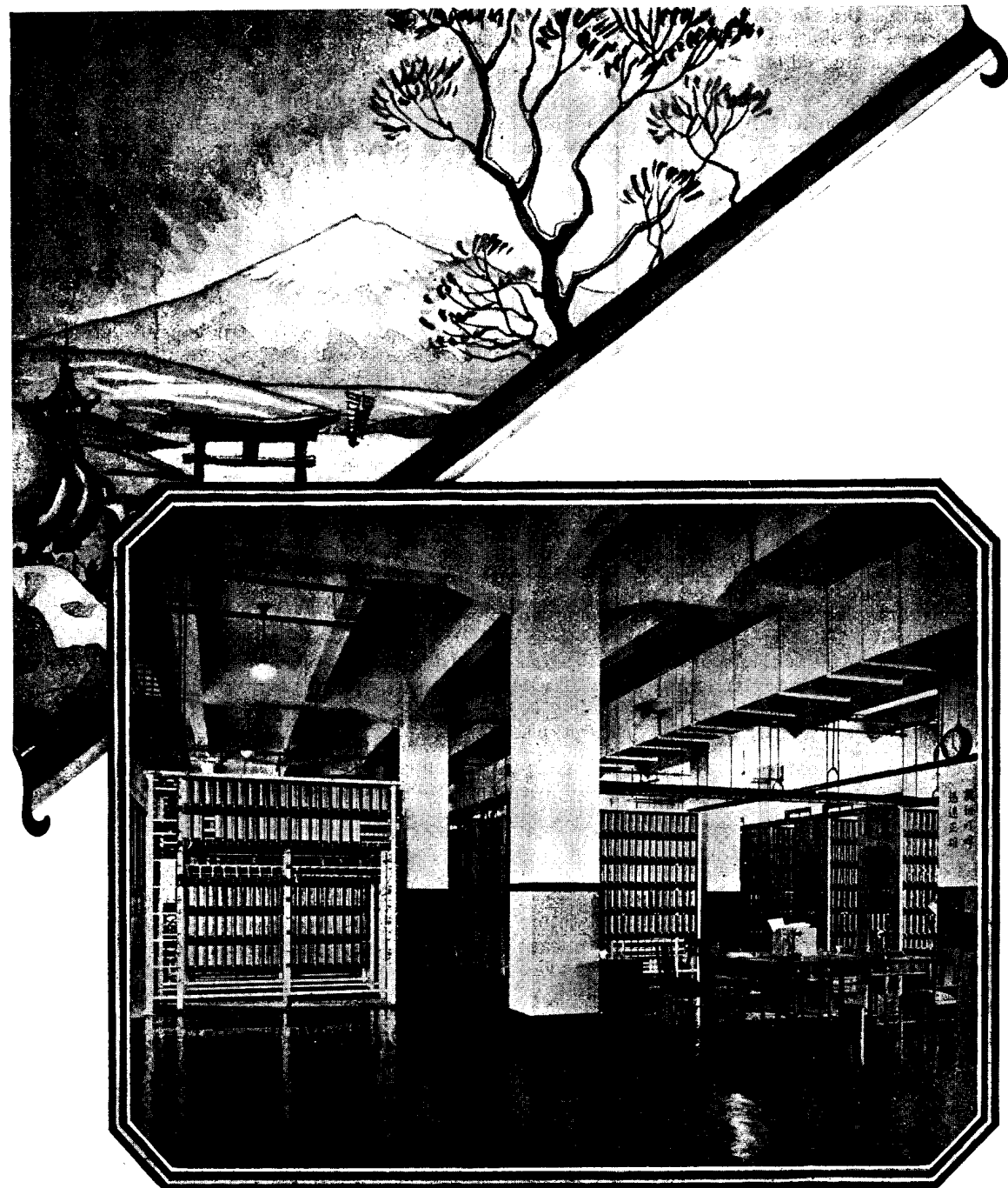
View of Strowger Automatic equipment at the Marunouchi Office, Tokyo, Japan. Note the excellent construction of the building which is fire-proof and earthquake-proof, with high ceilings and unusual provisions for light and ventilation.
