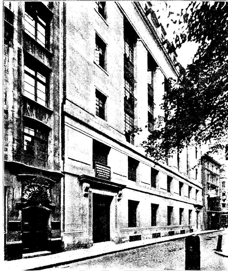
EXTERIOR OF METROPOLITAN AND NATIONAL EXCHANGES.
