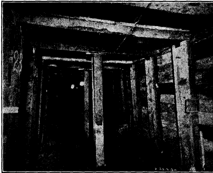
MAYFAIR—SUBWAY UNDER MOUNT STREET GARDENS.
