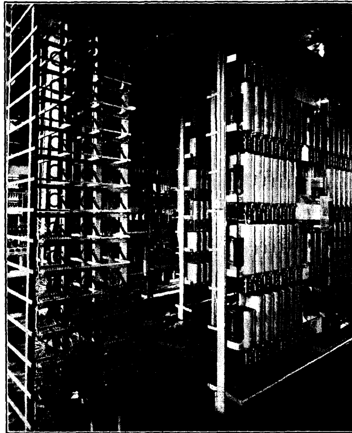
LONGFORD: TRUNK DISTRIBUTING FRAME AND FINAL SELECTOR RACKS.
