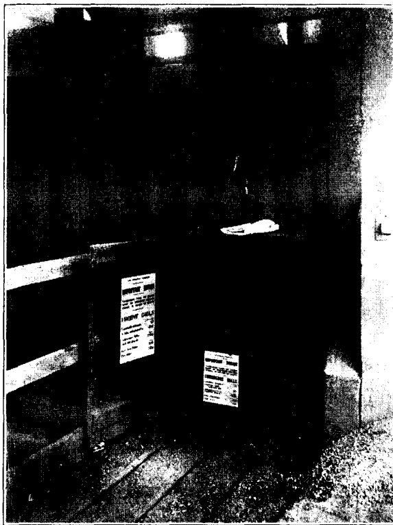
FIG. 1. PHONE AND CABLE HOUSED ON THE STAITH ALONGSIDE WHICH VESSEL IS BERTHED. NOTE WELL-USED TELEPHONE DIRECTORY.
