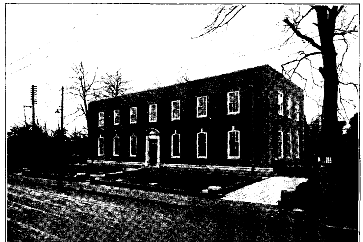
EXTERIOR VIEW OF ELMBRIDGE EXCHANGE.
