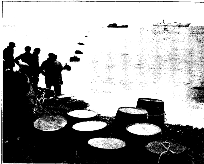
ANGLO-BELGIAN 1932 CABLE. LAYING A SHORE END.
