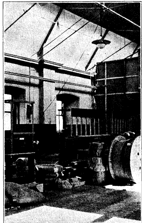
THE NEW TRUNK EXCHANGE, GLASGOW, IN COURSE OF CONSTRUCTION.
