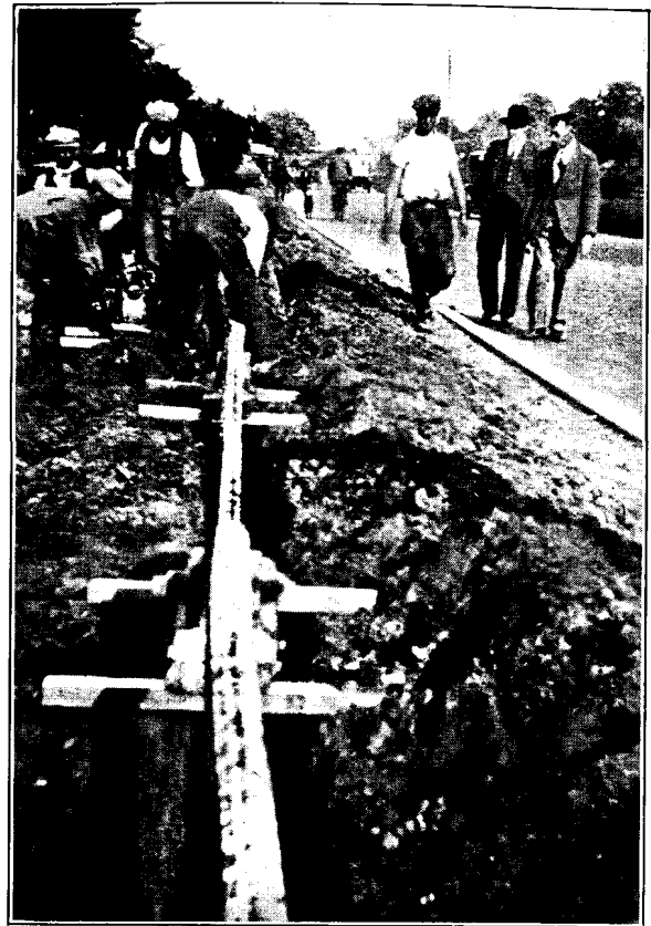
FIG. 4. PLACING 310 PAIR 25-LB. PLUS 4-SCREENED PAIR 40-LB. LEAD COVERED AND ARMOURD CABLE BETWEEN ASHFORD AND HYTHE.
