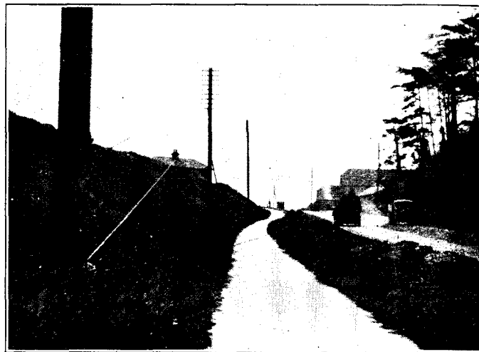
FIG. 2. LORRY DRAWING CABLE INTO POSITION.
