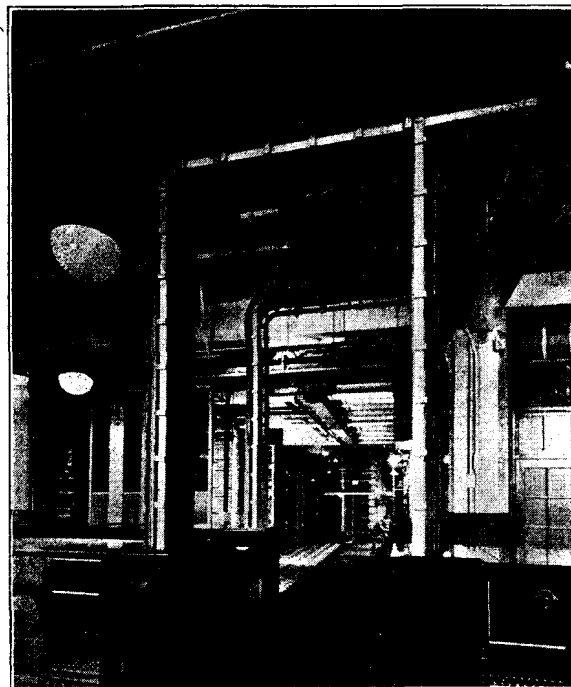
GENERAL VIEW OF SWITCHROOM, WITH TEST DESK IN FOREGROUND.
