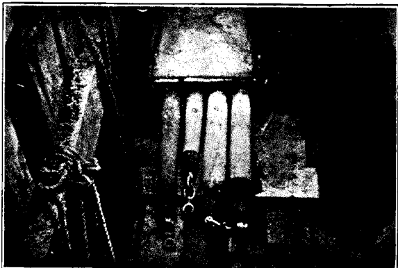
FIG. 14. RUBBER HOSE FORMERS SHOW PRESSURE TANK AND CLOSED ENDS WITH SECTION OF COMPLETE LAYER OF MULTIPLE DUCT.
