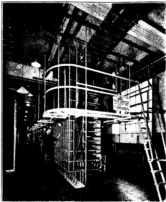
MAIN DISTRIBUTION FRAME.
