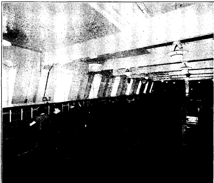
GENERAL VIEW OF AUTO-MANUAL SWITCHROOM.
