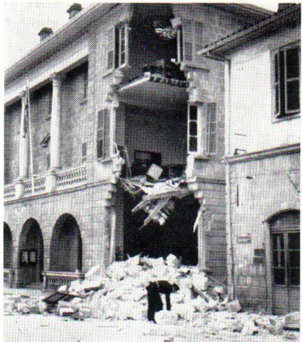
A time-bomb destroyed part of this post office building in Nicosia
