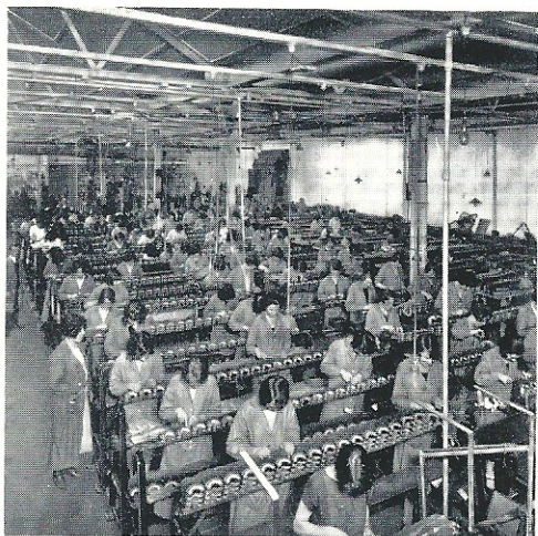
A Strowger Works flashback— wiring as it used to be
