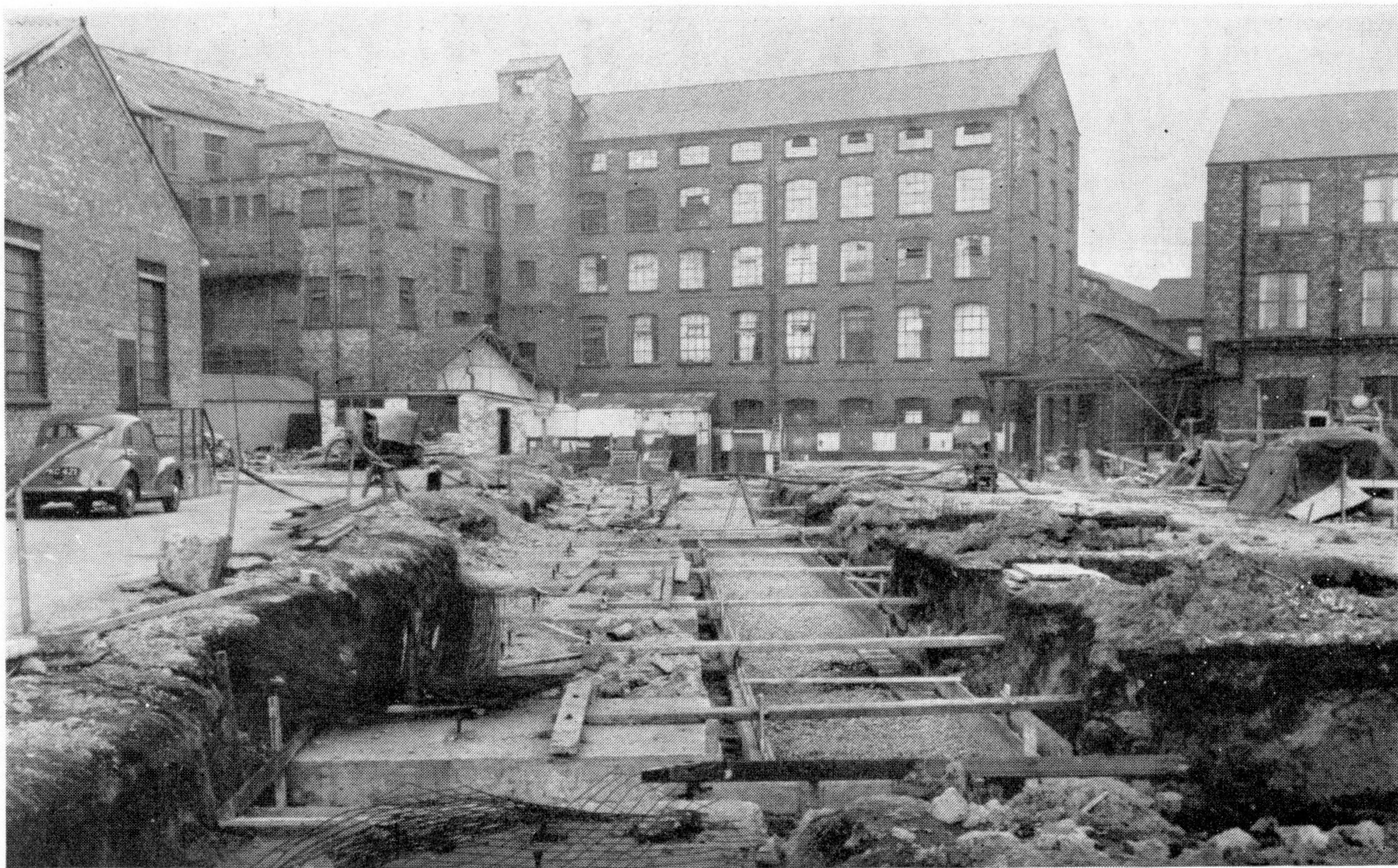
Shortly after the new multi-storey building was started. The site is being cleared and foundations are being laid
