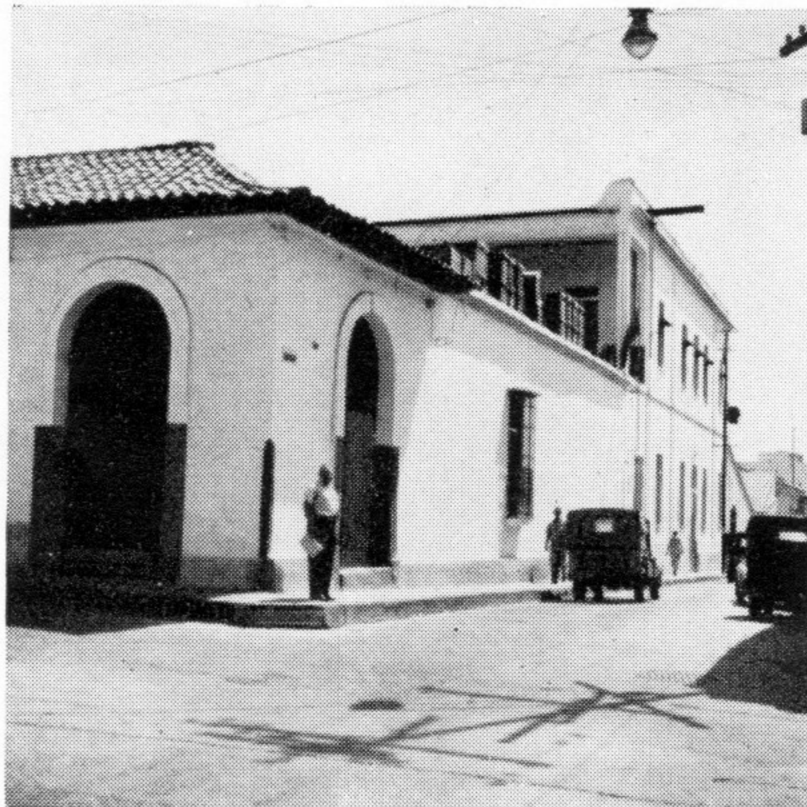
An exterior view of part of the Valencia exchange
