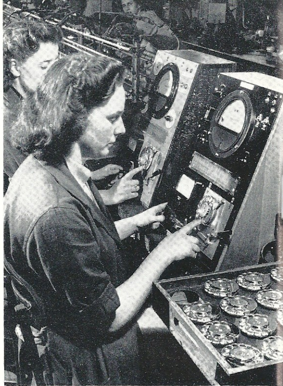
Automatic impulsing devices are used to test dials in Department 13
