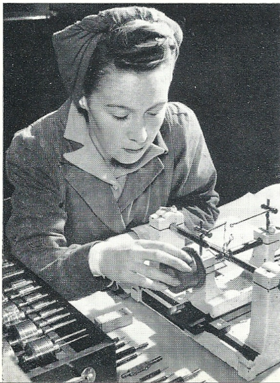
Measuring screw thread gauge in the Gauge Room
