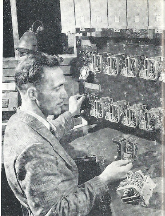
A stage in checking dial repeaters
