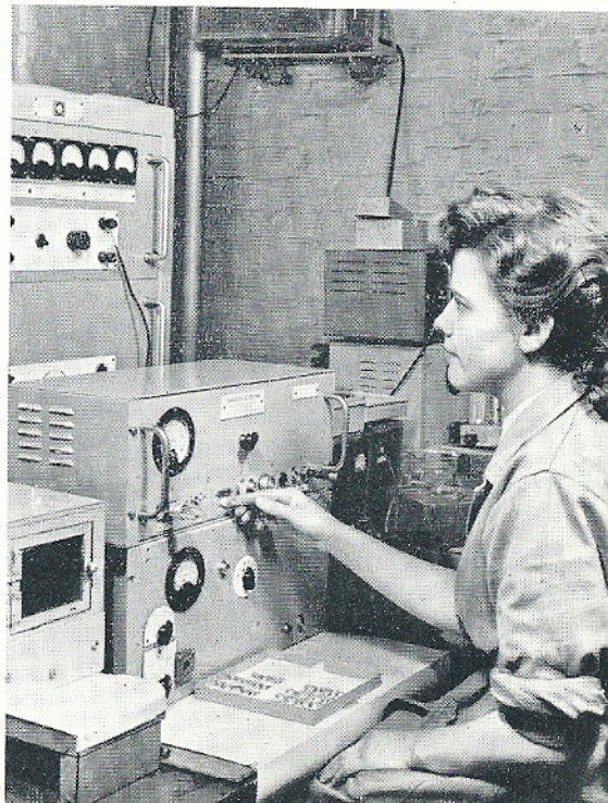
Checking frequency of a crystal
