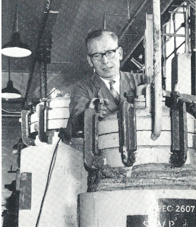
Muires Massey placing transformer coils in a vat for wax impregnation
