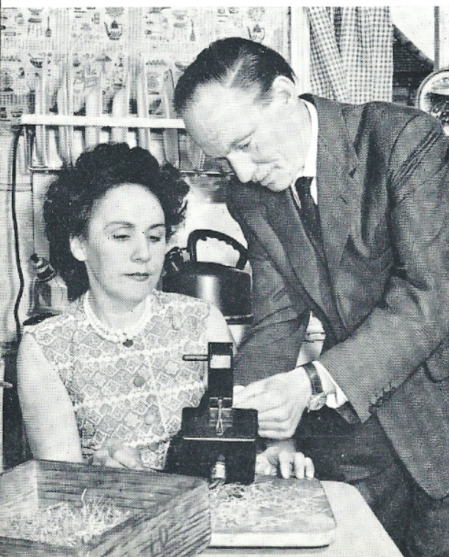
Rose learns how to test neon indicators
