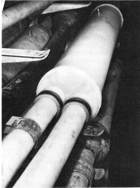
Fig. 1 Injection welded joint closure showing a 2 cable entry.
