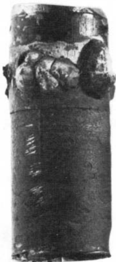
Figure 1. Corrosion of the Positive Pillar
