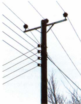
11 kV and 4V lines
