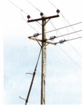
Tee-off pole, 3 phase 11kV line
