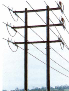
High Voltage systems come in various forms
