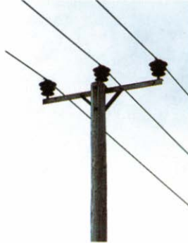
Single Circuit 3 phase 33kV line
