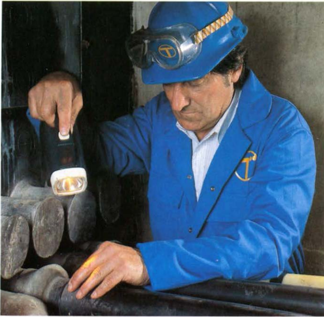
Ensure duct seals are in good condition.
