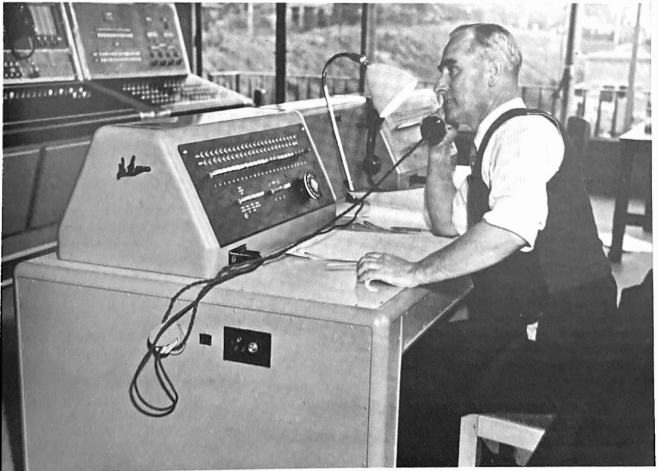
A telephone switchboard in use in Sandbach Signal Box
