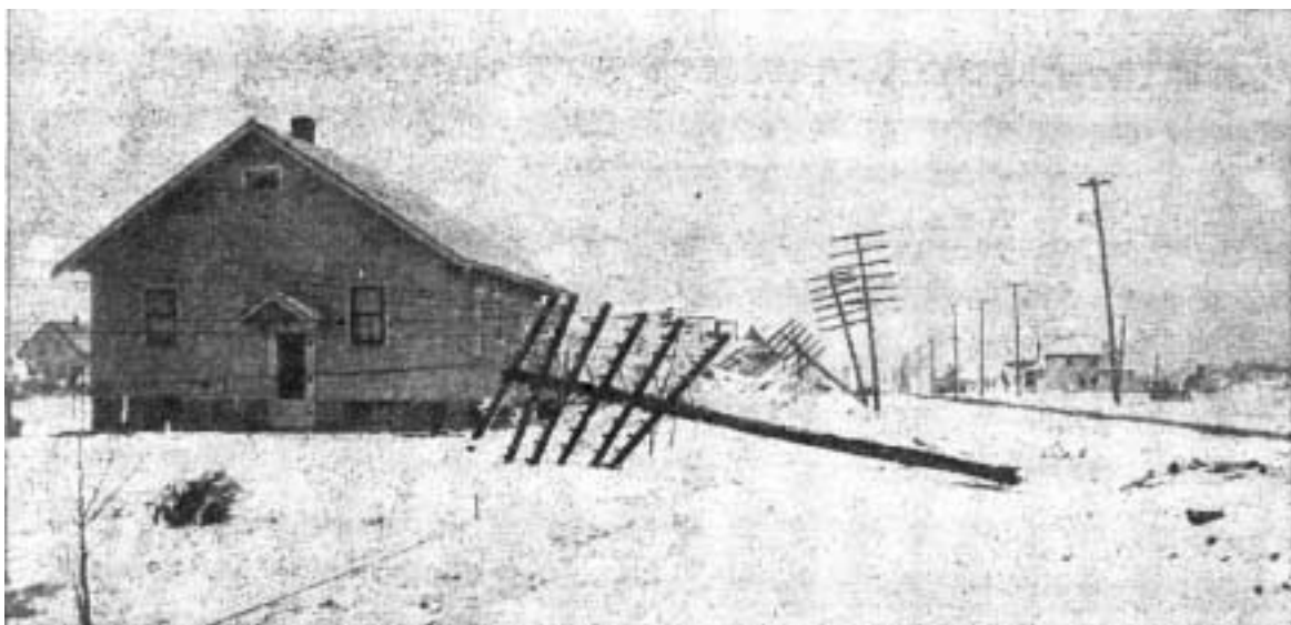
RADIO RESCUE. When 1930 blizzard downed hundreds of telegraph poles in North Dakota, Fargo-Bismarck radio hookup patched gap in NP dispatcher's line
