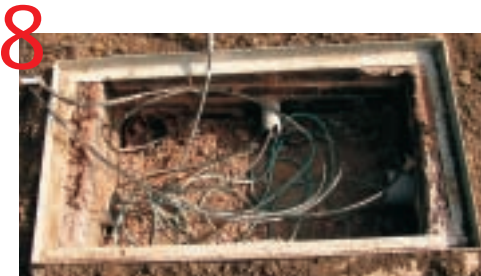
Unacceptable standard of finished box
