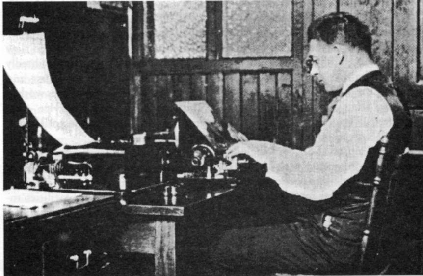
*R. Royan, the author of this article, at the opening in 1928 of one of the first Canadian Press printer circuits, between Toronto and Peterboro, Ontario. The Keyboard Transmitter is one of the original machines of its type made by the company. The Page Printer is a model 2P. These machines replaced the manual ones Morse operators formerly employed.*
